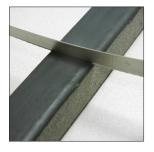
With a plastic spatula or trowel\* turn in the edges of the silicone face so that they remain snug and do not allow for the foam to be exposed. (\*metal tools could scratch the substrate).
